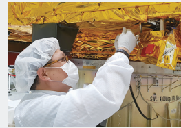
3 GK2A KSEM FM MLI Installation
